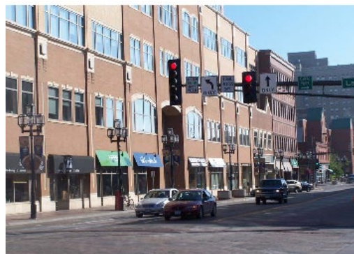
Example of Main Street Building III
