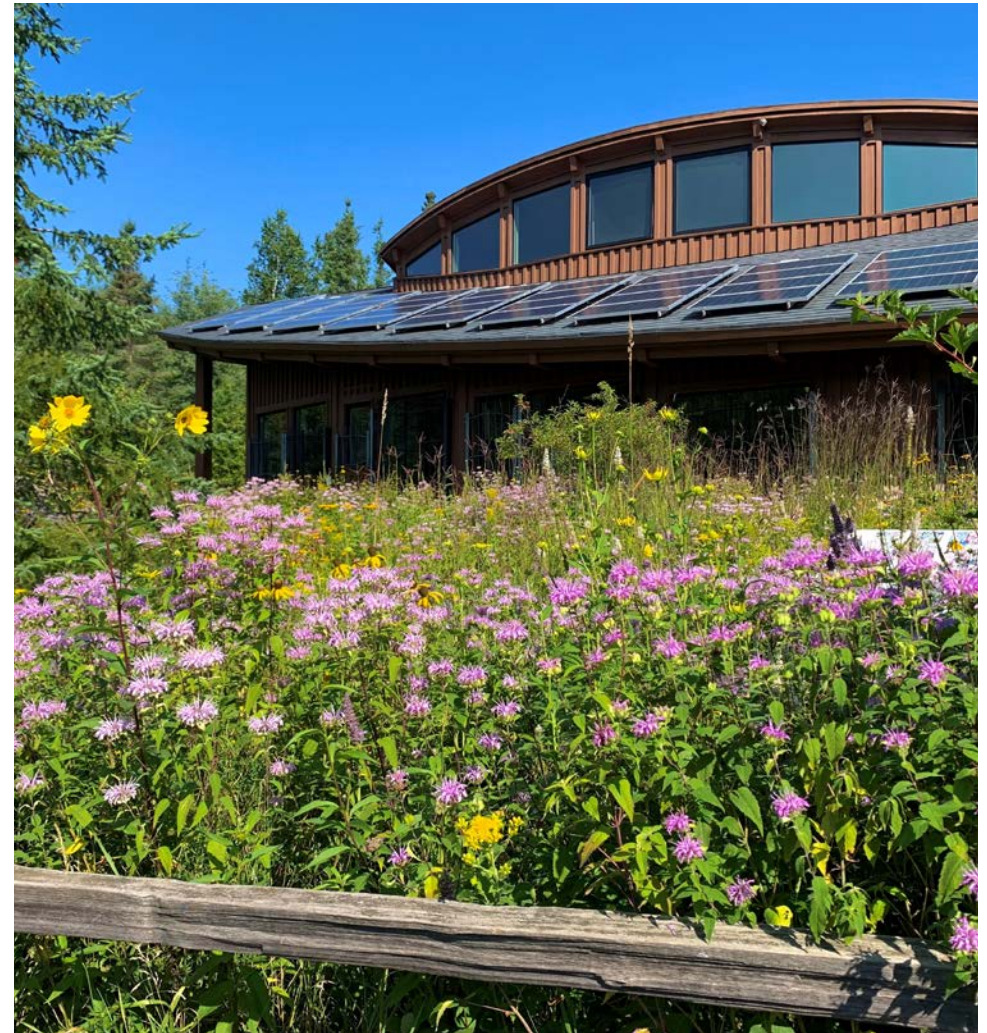
The Hartley Nature Center provides a strong example of opportunities to integrate climate resilience in design, such as incorporating solar panels, native pollinator habitats, and extensive stormwater management practices.
