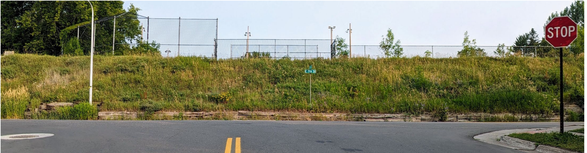
VIEW FROM NORTH 4 TH AVENUE EAST OF THE RETAINING WALL AND HILLSIDE SEPARATING EAST 7 TH STREET FROM FUTURE HILLSIDE SPORT COURT PARK AMENITIES
