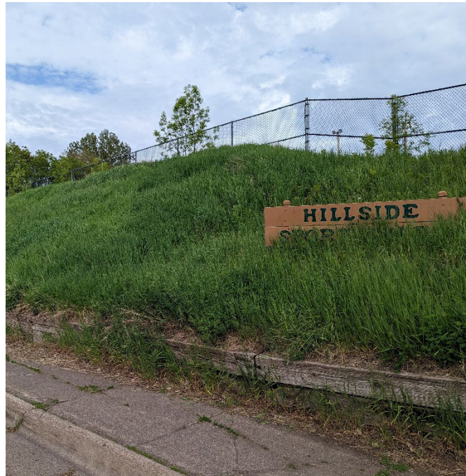
TIMBER RETAINING WALL AND ENTRANCE SIGN AT HILLSIDE SPORT COURT PARK (2023)
