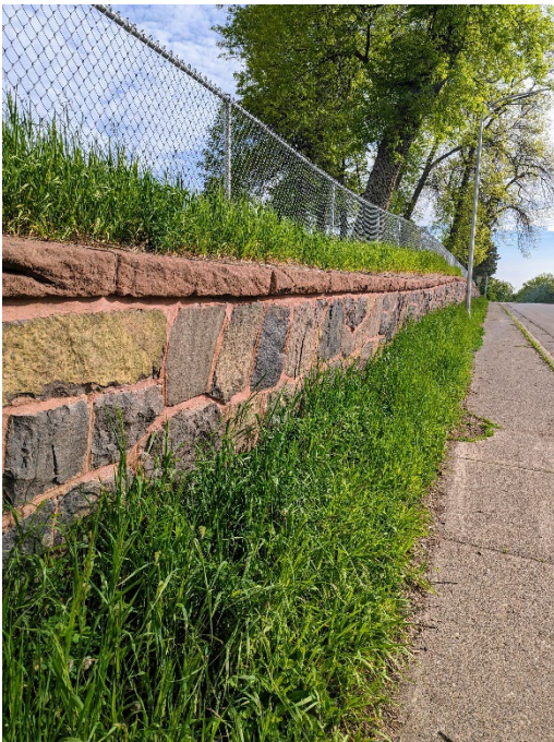
STONE RETAINING WALL AT HILLSIDE SPORT COURT PARK (2023)
