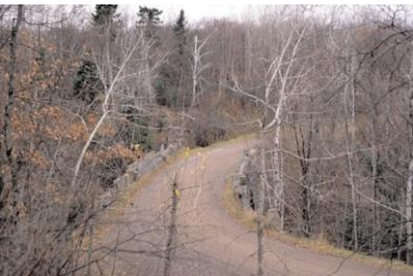
Stewart Creek bridge in late Fall.
