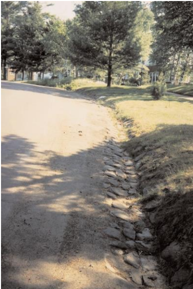
Stone gutters in Enger Park are an example of small-scale contributing structures of historic value.
