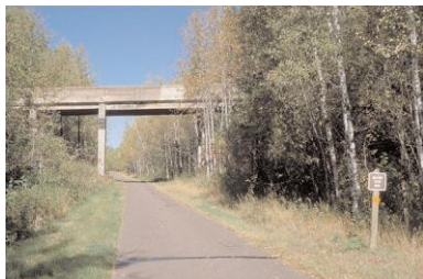
The Munger Trail passes under the Mission Creek trail segment.
