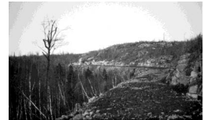
Bardon's Peak segment under construction in the 1920s. Photo: F. Rodney Paine.
