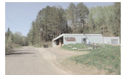
The Lakeview Sports Arena hockey rink is an example of a recreational structure not compatible with the historical integrity of Seven Bridges Road.
