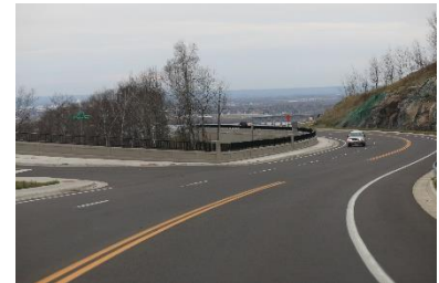
The reconstructed Haines Road intersection
