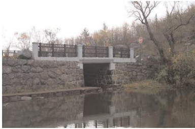
The Twin Ponds bridge.
