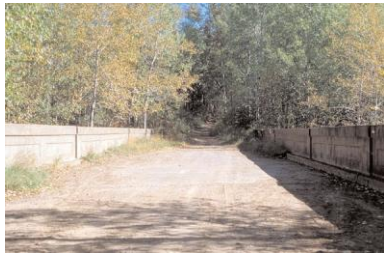
The railroad bridge carries the Mission Creek segment over the Munger Trail.
