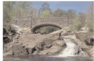
Bridge over Amity Creek on the Seven Bridges segment.
