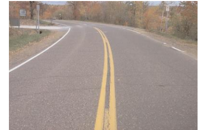
Bicycle lanes and pedestrian paths are lacking in many high use areas.
