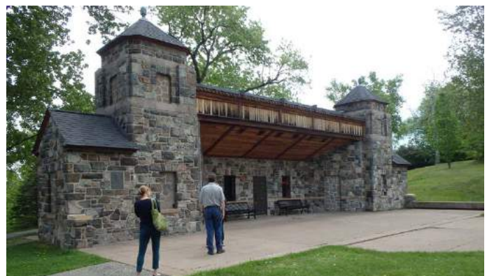
No operational restroom facilities in pavilion building
