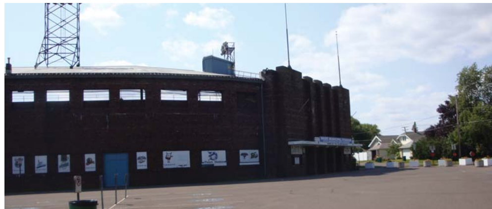
Wade Stadium entrance (prior to entry plaza construction)
