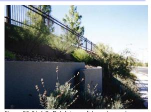
Figure 50-26.4-B: Retaining wall terracing and articulation
