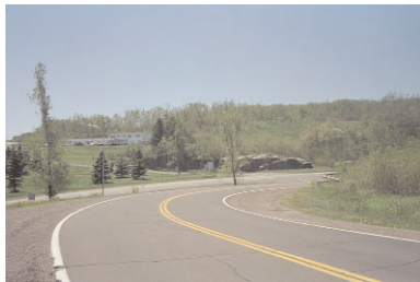
Modernized parkway segment near Highway 2
