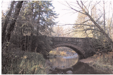
Historic bridge #4 on the Seven Bridges segment.
