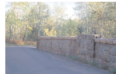
Native stone is used along the entire parkway in bridge and wall construction.
