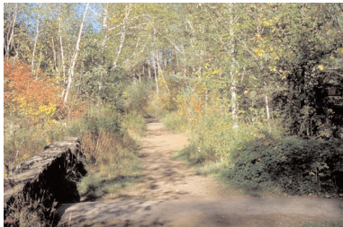
Can bridges along trail segments such as Amity Creek be restored?
