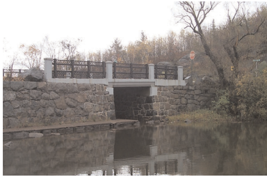
The Twin Ponds bridge.
