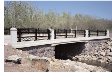
The new Keene Creek Bridge
