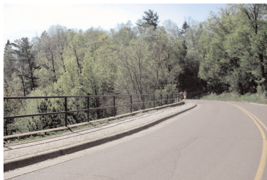
Narrow sidewalk along the Parkway at Chester Bowl, an area heavily used by pedestrians.
