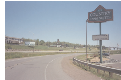
The Parkway near Boundary Avenue functions as a frontage road for I-35 with highway-oriented commercial services and signage.
