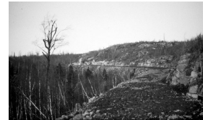
Bardon's Peak segment under construction in the 1920s. Photo: F. Rodney Paine.
