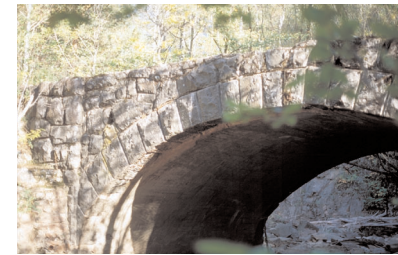
One of the stone-faced concrete arch bridges on the Amity Creek trail segment.
