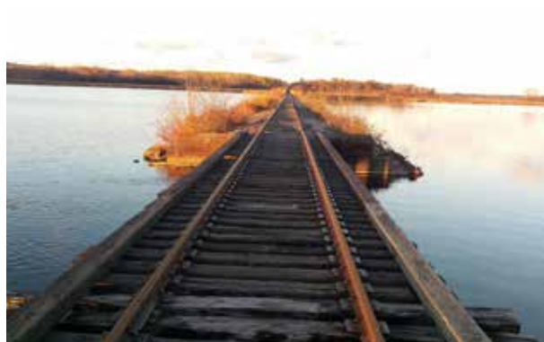
Figure 1.17 Segment 4 Existing Conditions
