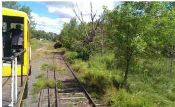
Figure 1.13 Segment 1 Existing Conditions
