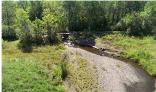
Figure 1.11 Existing Trail Crossing at Kingsbury Creek (future connection to Zoo)
