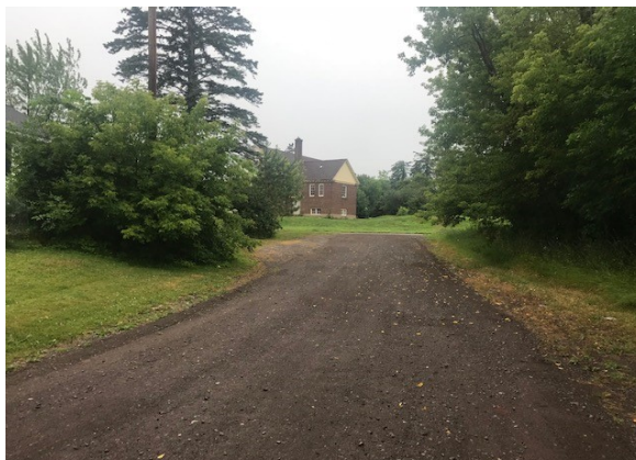
Parcel B parking area facing north
