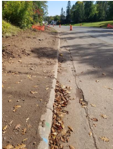
Construction sediment at MS-5
