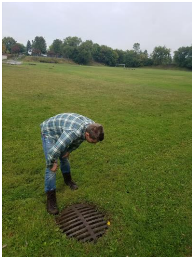
Catch basin at soccer field
