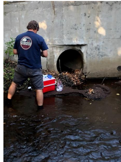
Storm drain outfall at MS-5
