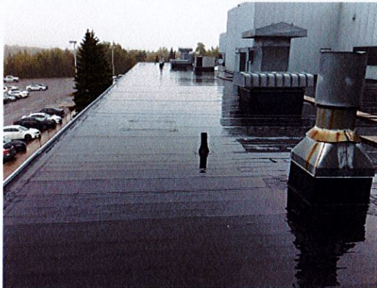
Section Overview Several areas of siding are still in need of replacement on this level
