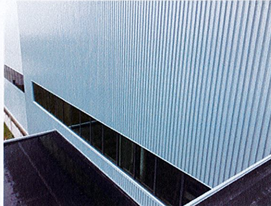
New wall panels have been installed
