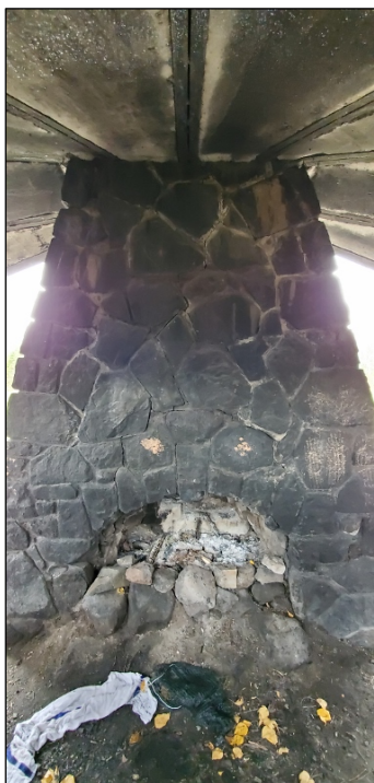
Photograph 4. SL-DUL-3132, October 2019, interior view of chimney, looking northwest
