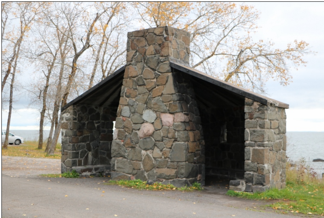
Photograph 1. SL-DUL-3132, October 2019, looking northeast
