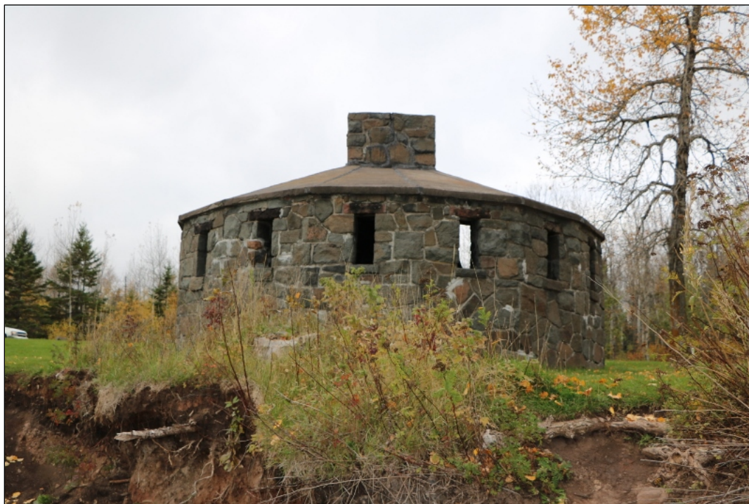
Photograph 3. SL-DUL-3132, October 2019, looking northwest
