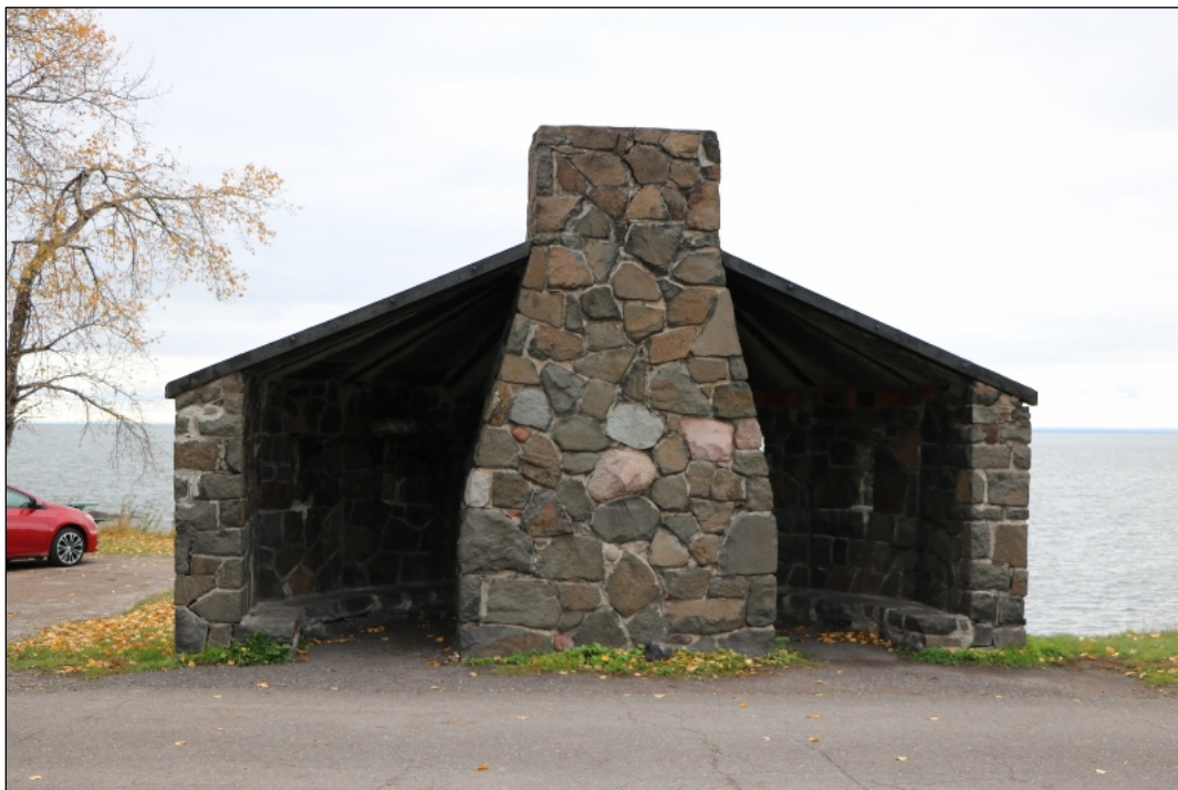
Photograph 2. SL-DUL-3132, October 2019, looking east
