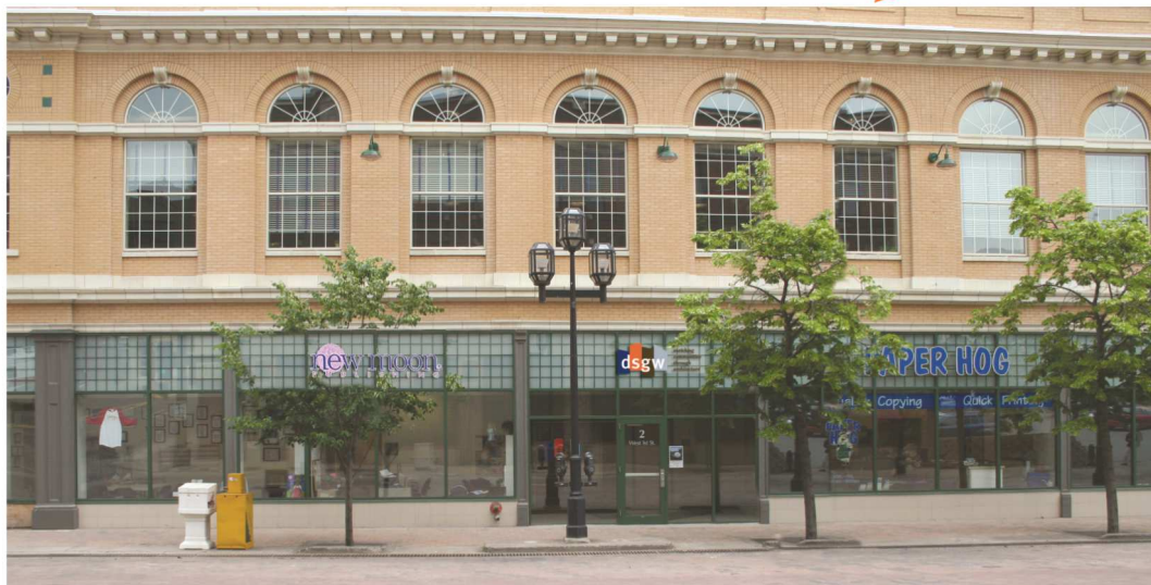
Example of Storefront Window
