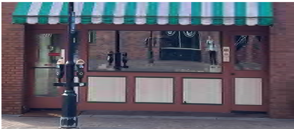
Photograph 20: View of painted storefront within the historic district.
