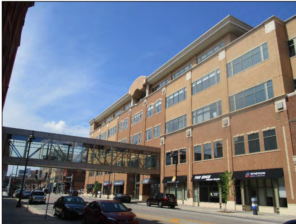
13 East Superior Street (Non-historic infill)
