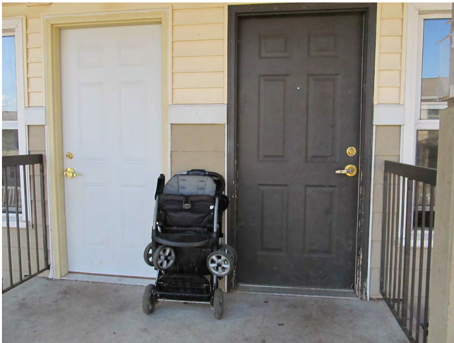
Figure 8 Mix of door ages and conditions. Dented on right, new on left.
