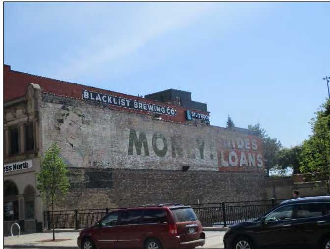
Photograph 26: Historic walls signs, like this example of a painted sign, should be preserved, however painting previously unpainted brick should be avoided.
