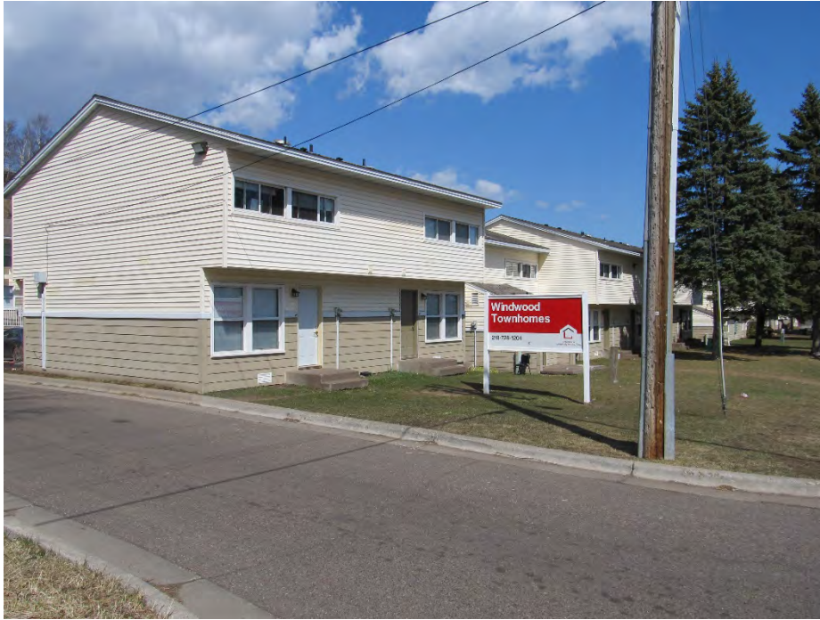
Figure 1 View of complex from road.
