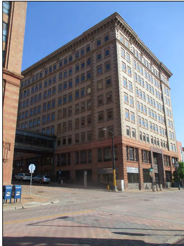
225-231 West 1st Street (Historic Name: Wolvin Building)
