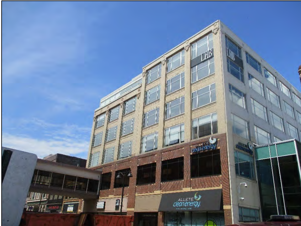
Photograph 4: View of two industrial vernacular buildings at 17-23 W. Superior Street. The buildings originally held a furniture warehouse and a dry goods warehouse. Note the large window openings and lack of architectural ornament below the cornice level.
