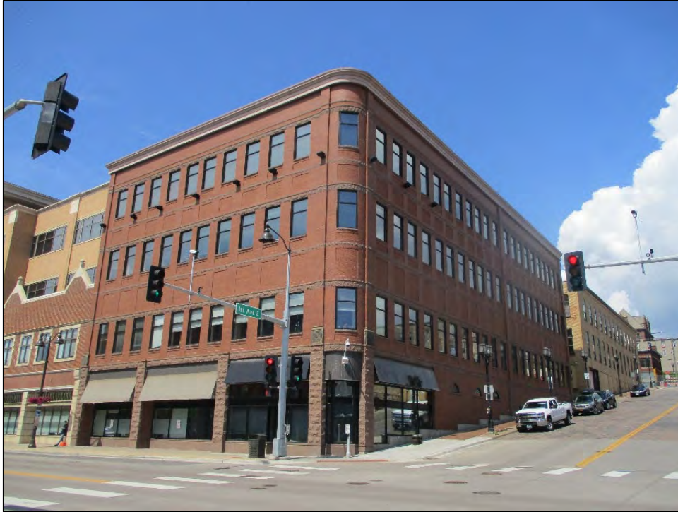
13 East Superior Street (Non-historic infill)
