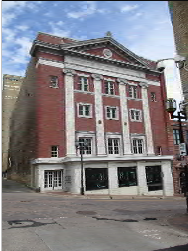
Photograph 5: View of the Classical Revival Orpheum Theatre on N. 2 nd Avenue E. Note the pediment, ionic pilasters, and keystone window lintels at the 3 rd story.
