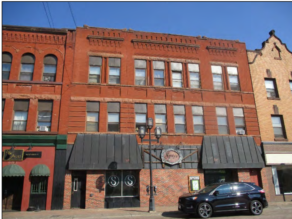
109-111 West 1st Street (Historic Name: New England Hotel)
