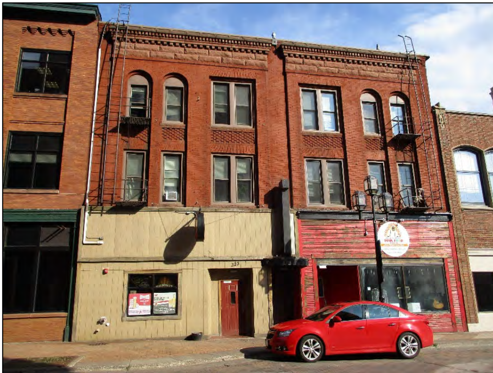
321-323 West 1st Street (Historic Name: Mason Flats)
