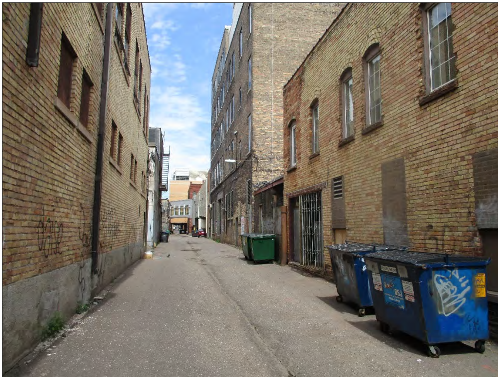
Photograph 33: View of alley within the historic district. Alleys can be used for support functions including storage of trash receptacles.
