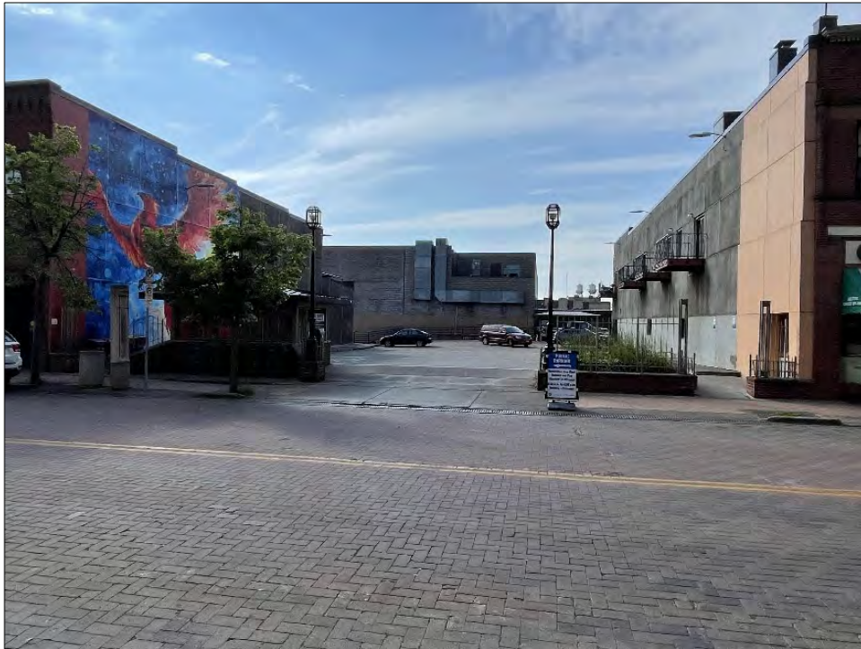
Photograph 36: View of parking lot within the historic district created by the past demolition of historic buildings.
