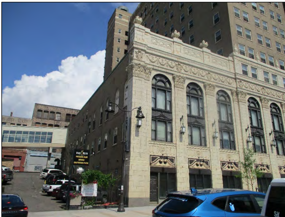
217 East Superior Street (Parking Lot)
