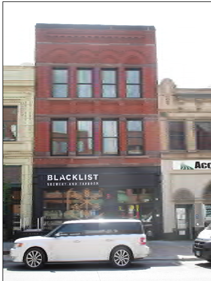
Photograph 7: View of the Italianate building at 120 E. Superior Street.
