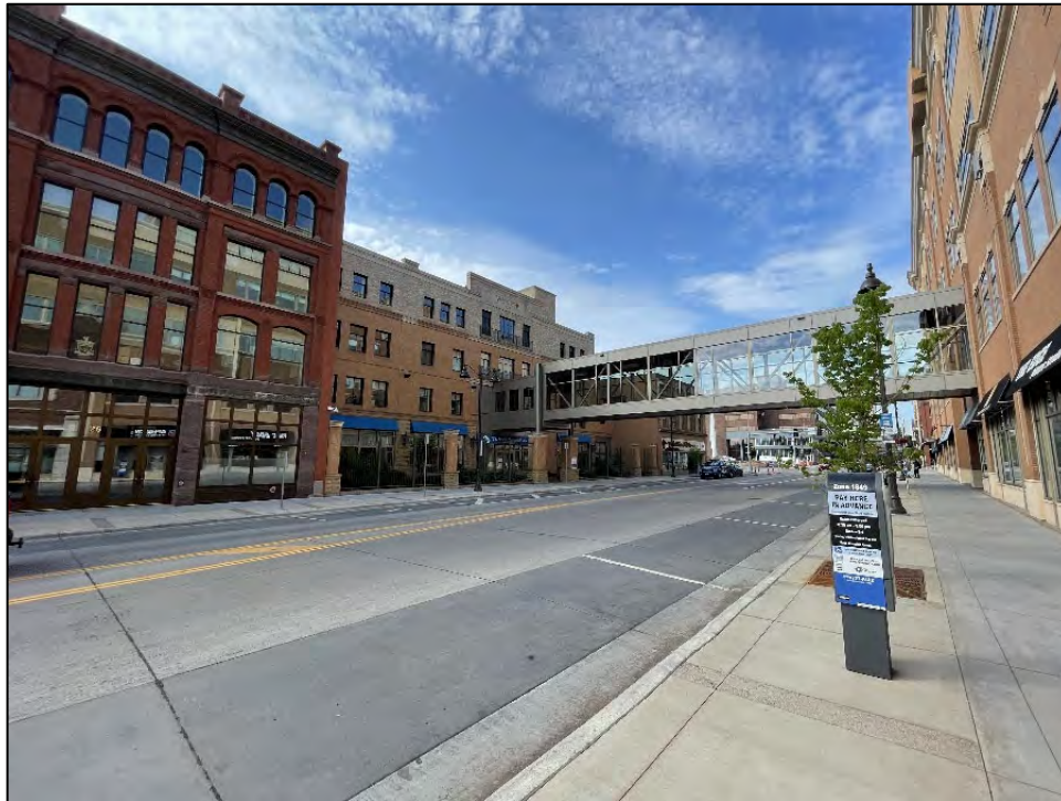
16-24 East Superior Street (Non-historic infill)
