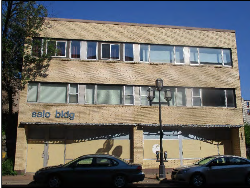
15-17 East 1st Street (Historic Name: Dunlap Building)
