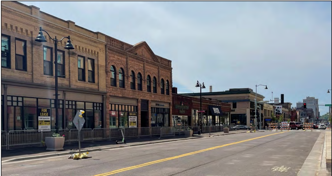
Photograph 11: View of the district along East Superior Street, looking towards East 3 rd Avenue.
