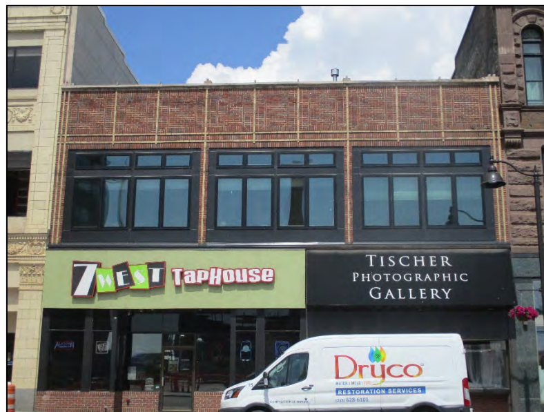
5-7 West Superior Street (Historic Name: Norris-MacDougal Block)
