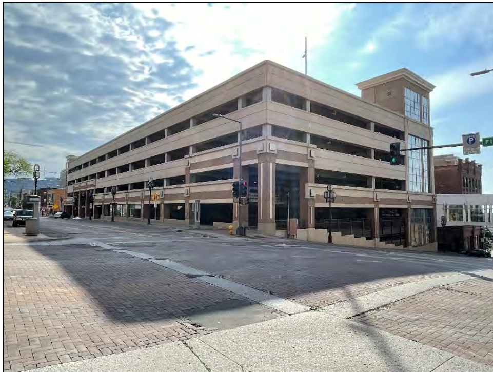
2-28 East 1st Street (US Bank Parking Garage)
