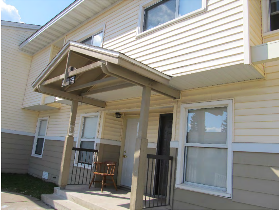
Figure 9 Porch system, generally in good condition
