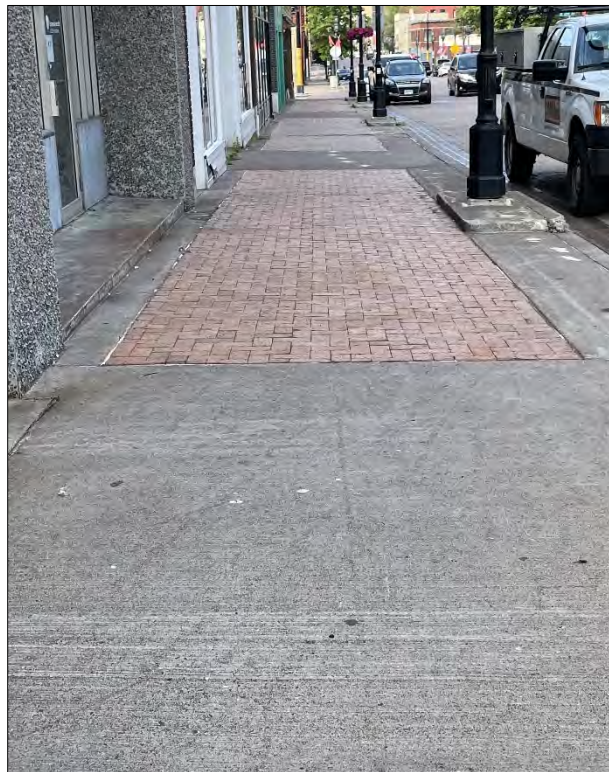
Photograph 38: View of 1985 brick sidewalk located within the historic district.
