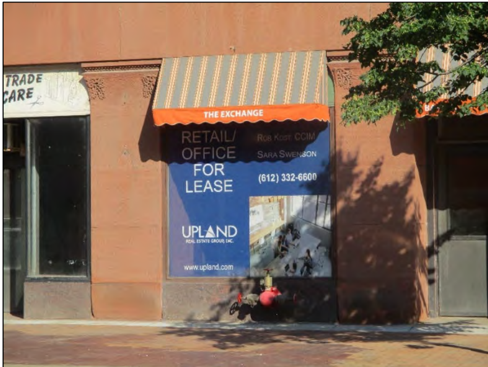
Photograph 28: Signs can be placed on the front flap of an awning or canopy as seen in this example located within the historic district.
