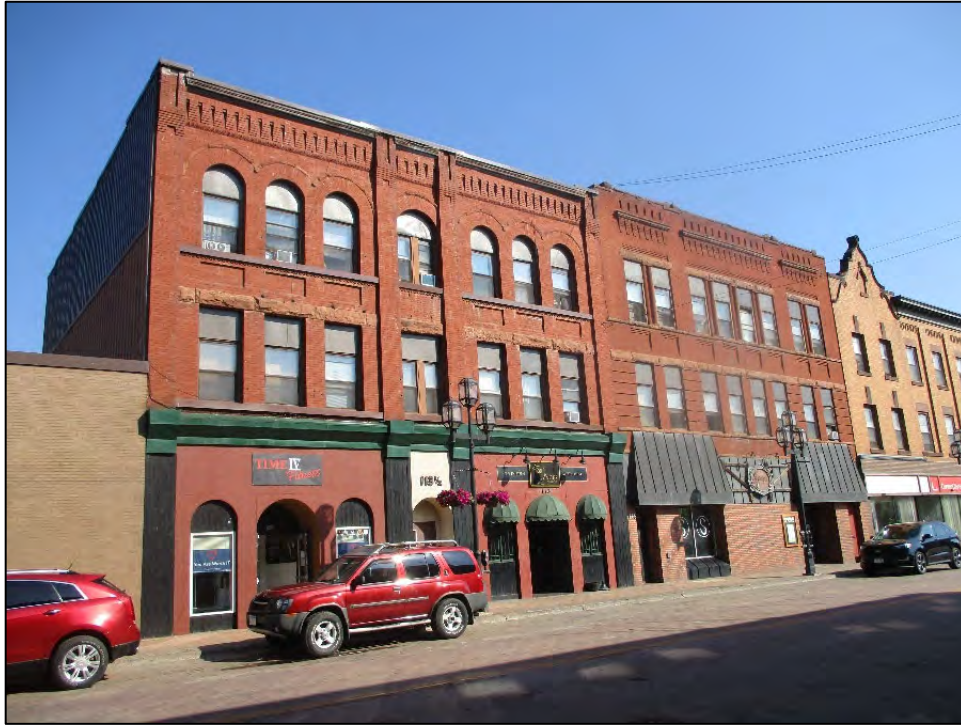
113-115 West 1st Street (Historic Name: Columbia Block)
