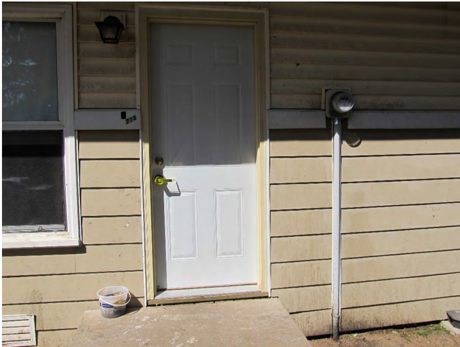
Figure 4 Lower fiber cement siding installed down to grade
