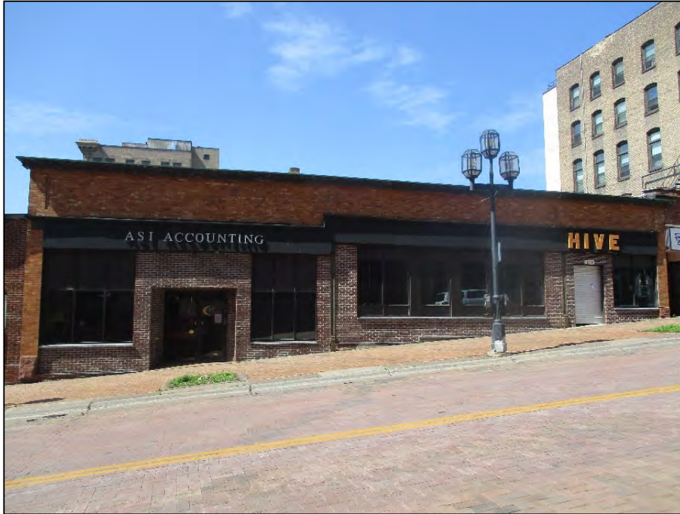
109 West 2nd Avenue (Historic Name: commercial building)
