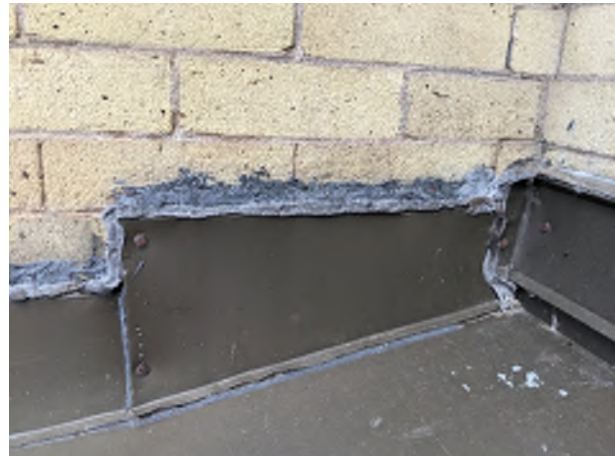
PICTURE #14 Roof/Wall Flashing
