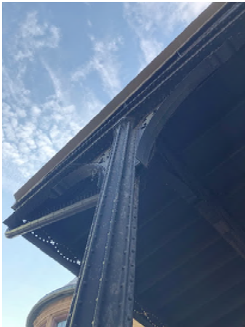
PICTURE #23 Roof/Wall Flashing
