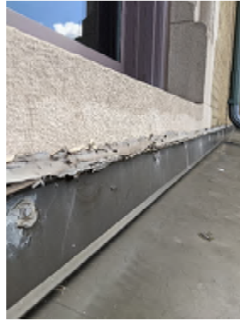
PICTURE #12 Roof/Sill Flashing
