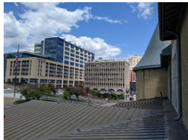
PICTURE #10 Roof Standing Seam
