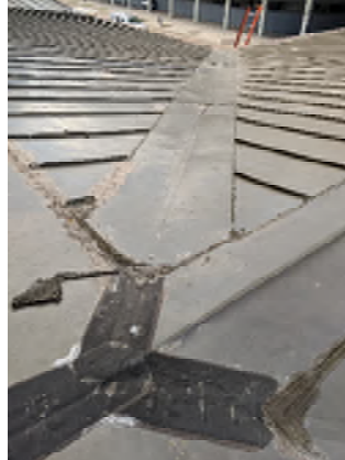
PICTURE #19 Roof Valley
