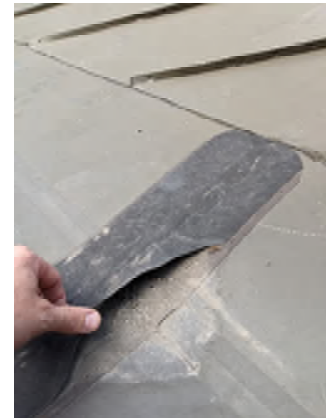
PICTURE #20 Roof Valley
