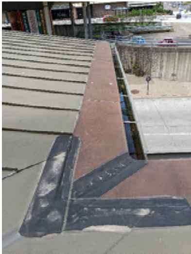
PICTURE #15 Roof Edge/Gutter
