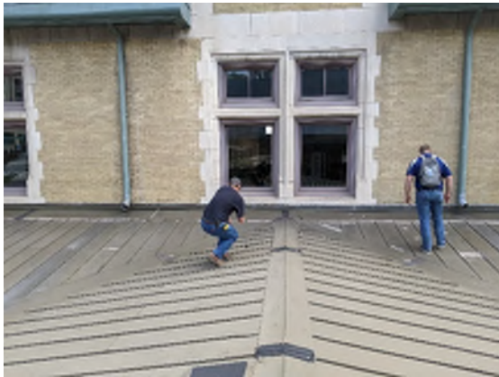
PICTURE #18 Roof Ridge
