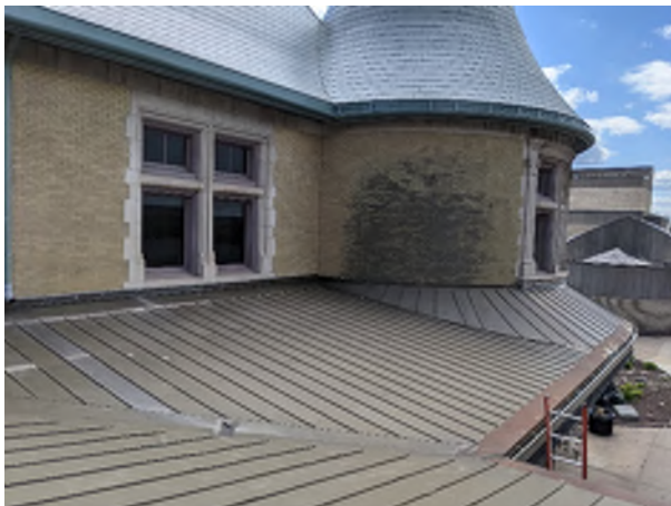
PICTURE #9 Roof Standing Seam
