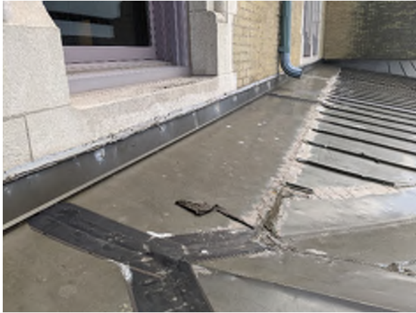
PICTURE #11 Roof/Sill Flashing
