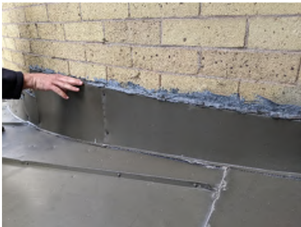
PICTURE #13 Roof/Wall Flashing
