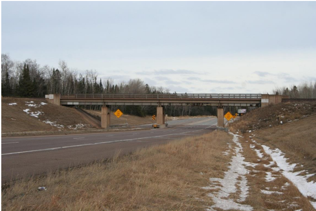
Figure 5. DM&IR railroad overpass bridge (Br. No. 38001; LK-THB-139) at the end of TH 61, near Two Harbors, view facing east.
