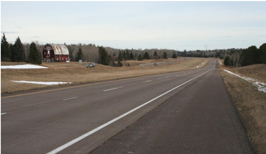
Figure 9. TH 61, near mile marker 15, view facing east. Note the barn to the rear left of the photograph. The trunk highway alignment bisected a number of existing farms and woodland areas.
