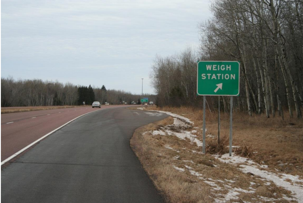
Figure 20. Weigh station pull-off located near Lakewood Drive and mile marker 8, view facing west. The weigh station pull-off was added c.1970.
