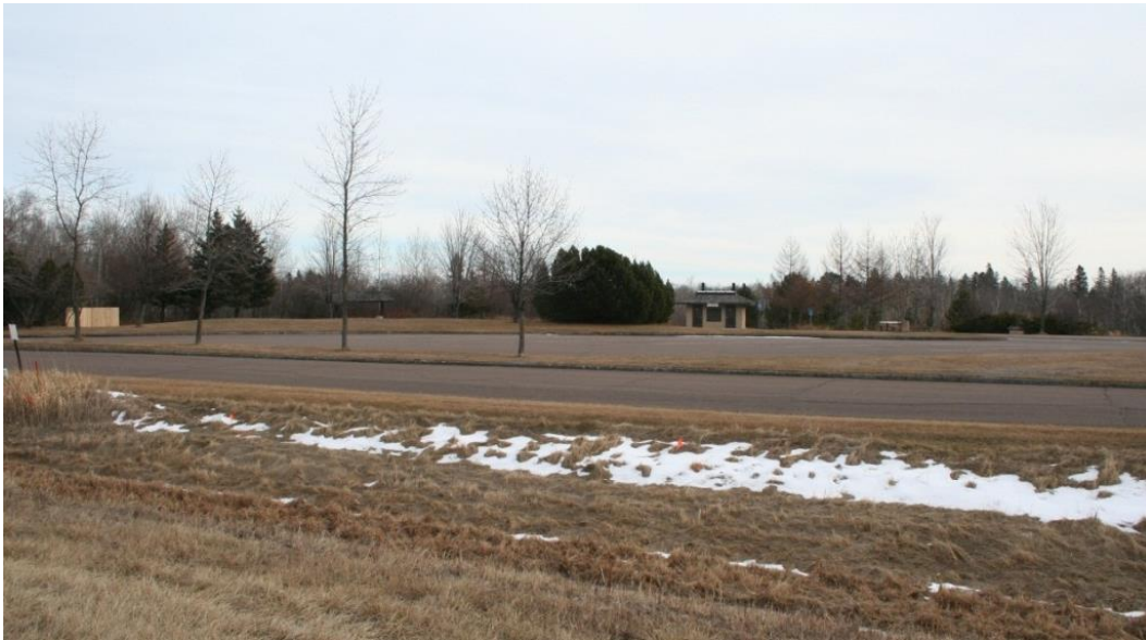
Figure 13. Knife River rest area (LK-UOG-031), located east of the Knife River, view facing southeast. Overview of the rest area parking area and restroom (constructed 1995).
