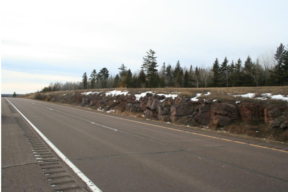
Figure 6. Detail of the elevation change between the northbound and southbound traffic between mile marker 18 and 19, view facing northwest.
