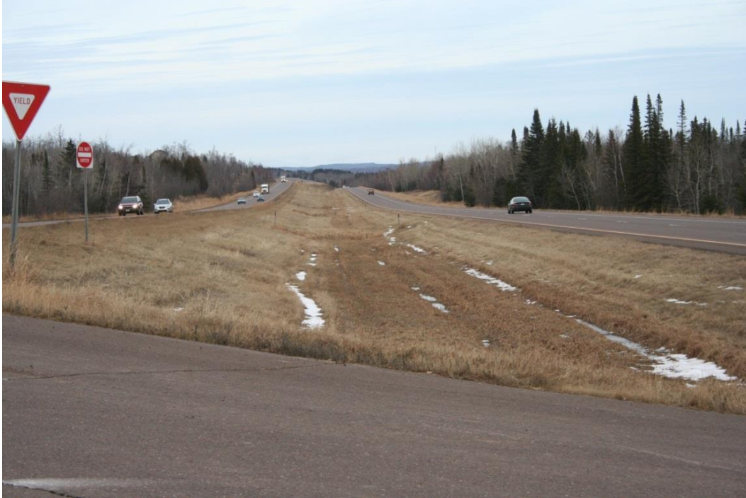
Figure 14. Typical median along TH 61, view facing east.
