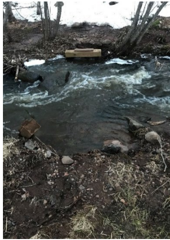
Hartley – Marshall Street entrance
